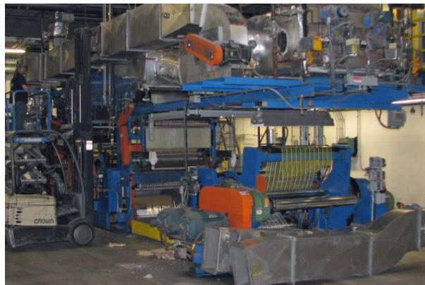
Dismantling the old Kidder Press.
